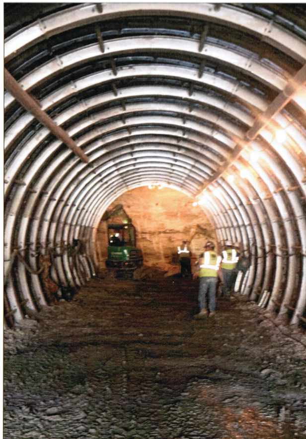
The tunnel as construction progresses beneath the roadway.
